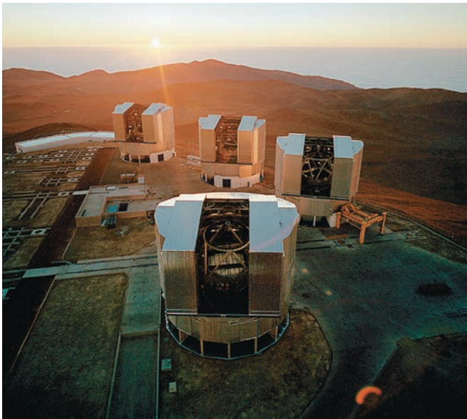
▲ FIGURE 5.11 VLT Observatory Located at the Paranal Observatory in Atacama, Chile, the European Southern Observatory's Very Large Telescope (VLT) is currently the world's largest optical telescope. Four 8.2-m reflecting telescopes are used in tandem to create the effective area of a single 16-m mirror. (ESO)
