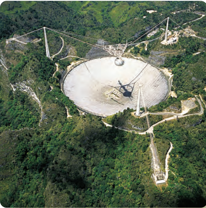
▲ Figure 6-17 The 305-m (1000-ft) radio telescope in Arecibo, Puerto Rico, is nestled in a naturally bowl-shaped valley. The receiver platform is suspended over the dish. A consortium led by SRI International and Universities Space Research Association (USRA) manages Arecibo Observatory for the National Science Foundation (NSF).
